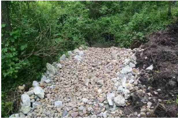
PROPOSED ROCK BEACHED PLACEMENT STYLE NOT TO SCALE
